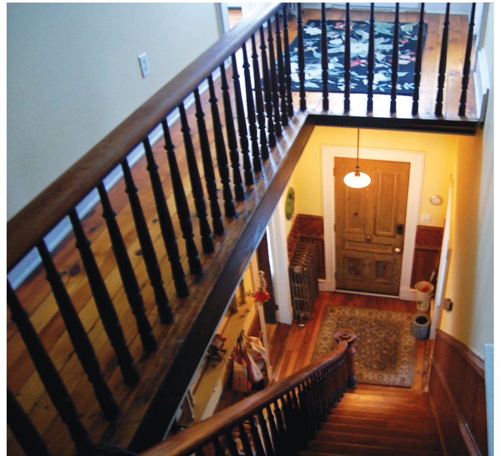
Months of careful restoration brought the original staircase back to its original glory.
